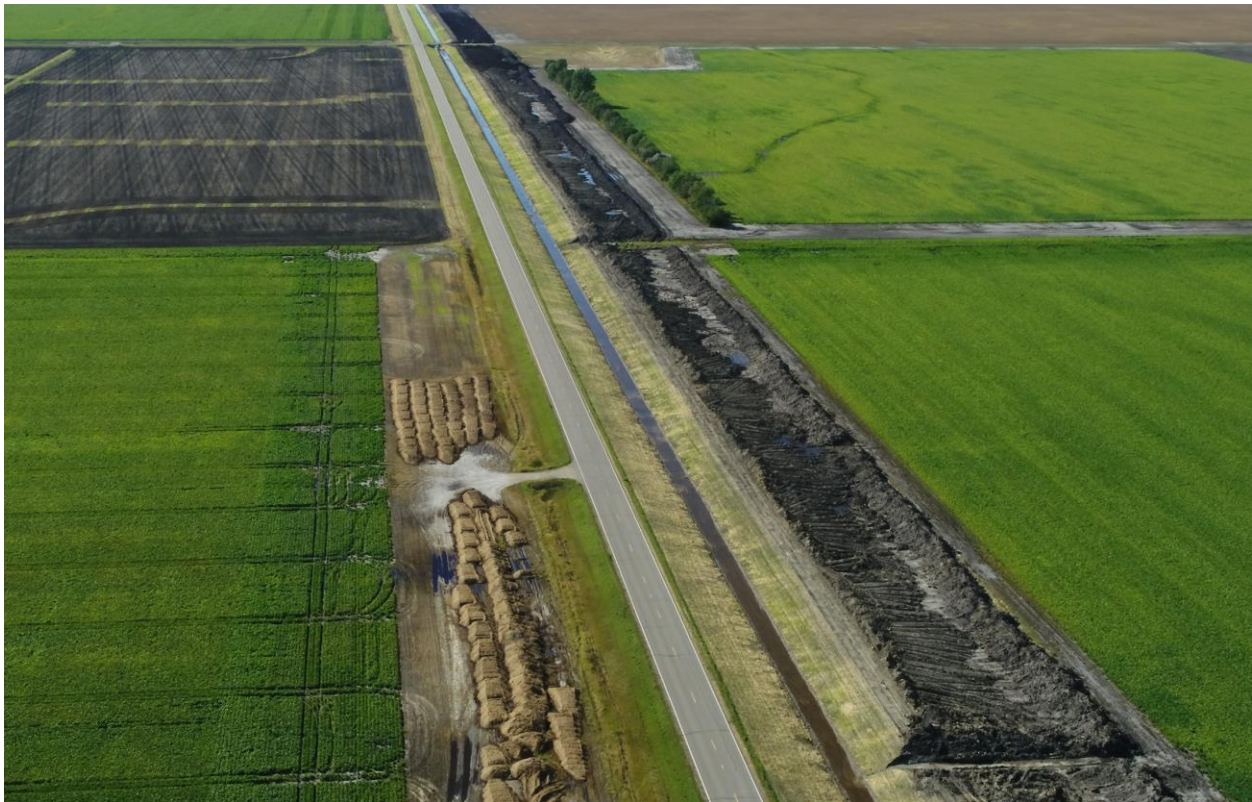
Ditch Retrofits provide significant progress to many of the Joint Comprehensive Watershed Management Plan goals.
