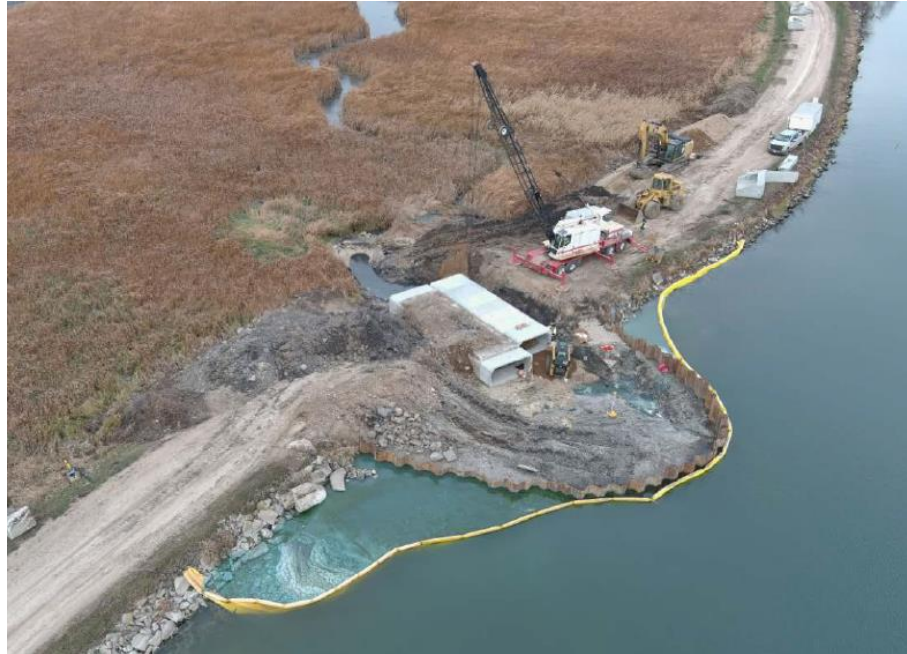
Lightning Lake Outlet Project No. 1 Granular Fill Placement
