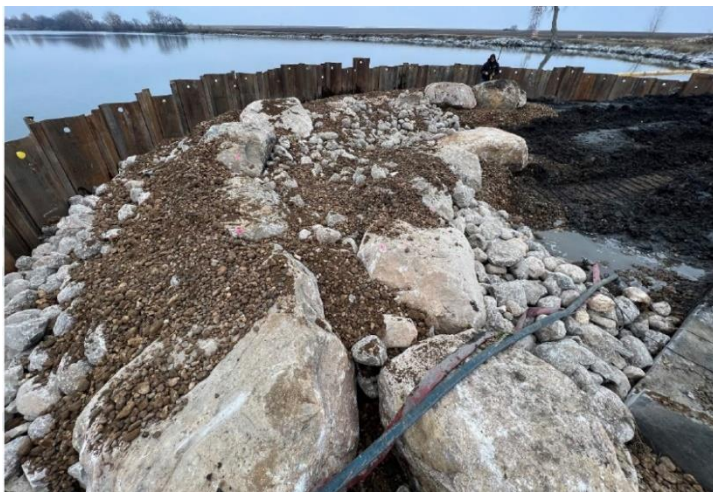
Lightning Lake Outlet Project No. 1 Boulder Weir Placement
